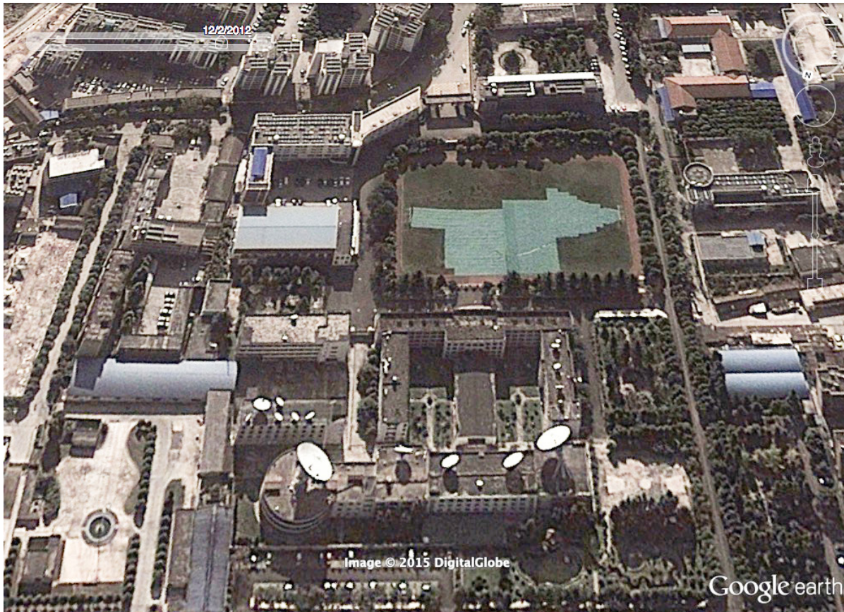
Figure 3: PLA Chengdu MR 2nd TRB MUCD 78020; 158 Jiaochang East Road, Wuhua District, Kunming (云南省昆明市五华区教场东路158号); Image by Digital Globe, via Google Earth. Date of image: 12/2/2012.
